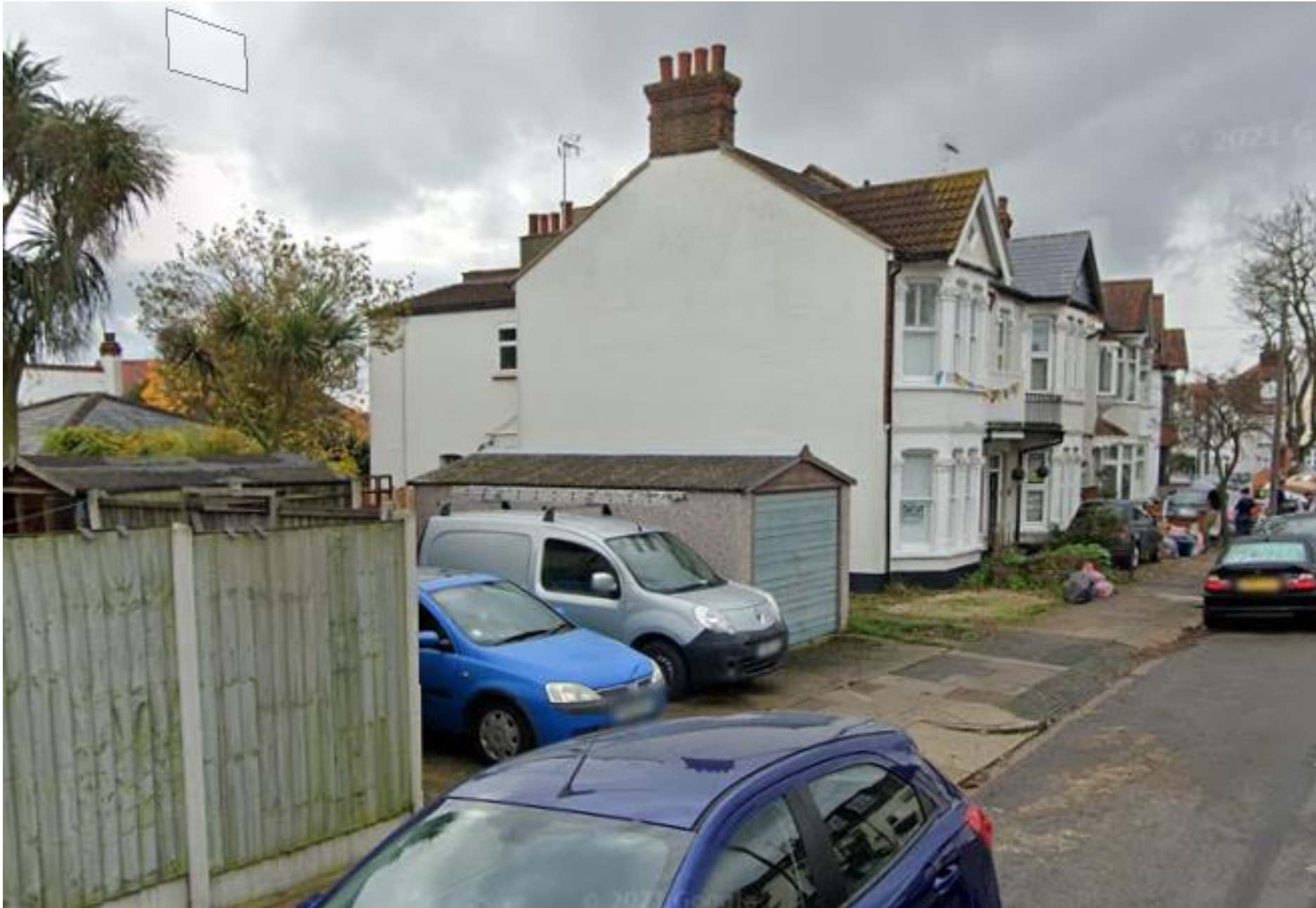
View of the front, side and rear of 8 Somerville Gardens from the public highway prior to development in 2020.
