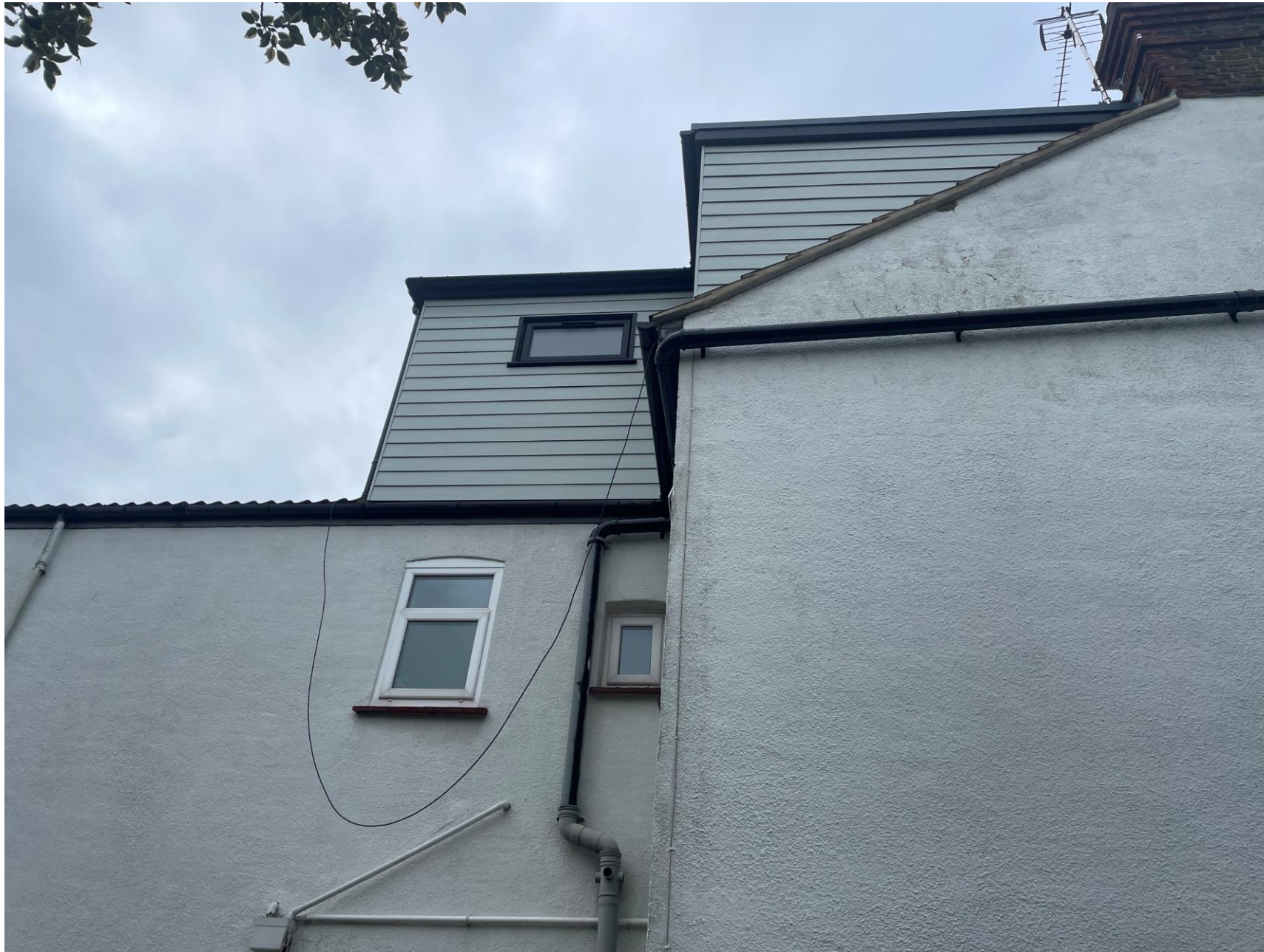
The dormer from the side of No. 8 Somerville Gardens
